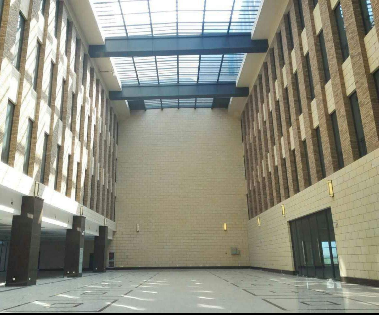
MCM SANDSTONE INTERIOR CLADDING
